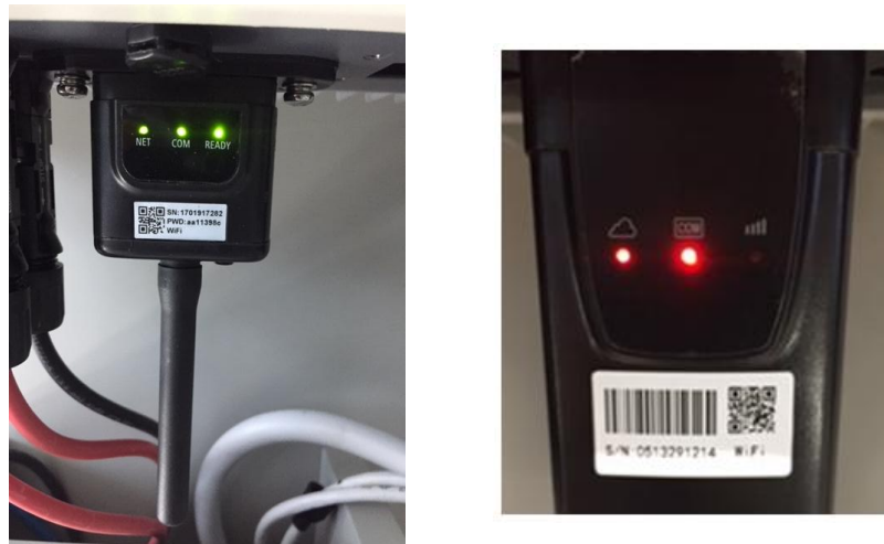
Figure 102 - Final status of LEDs
