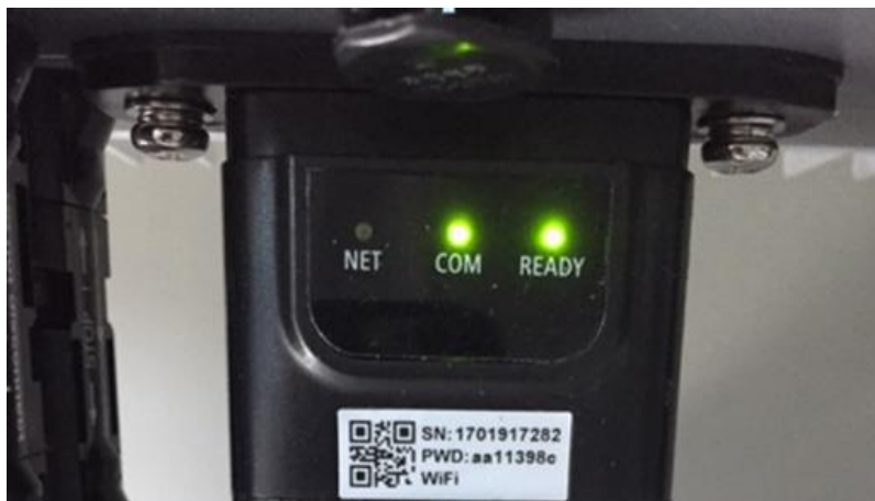
Figure 113 - Initial status of LEDs
