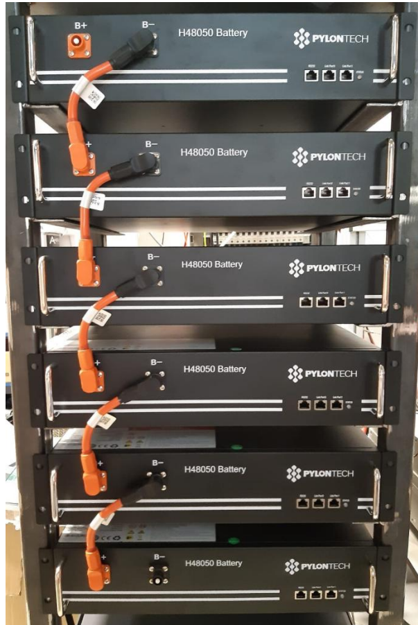
Figure 18 - Power cable between battery modules
