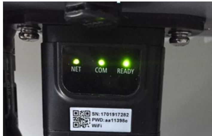
Figure 114 - Final status of LEDs
