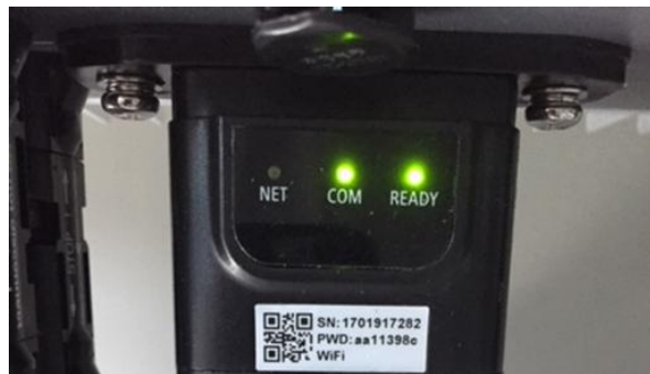
Figure 119 - Initial status of LEDs
