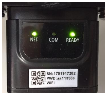
Figure 121 - Irregular communication status between inverter and adapter
