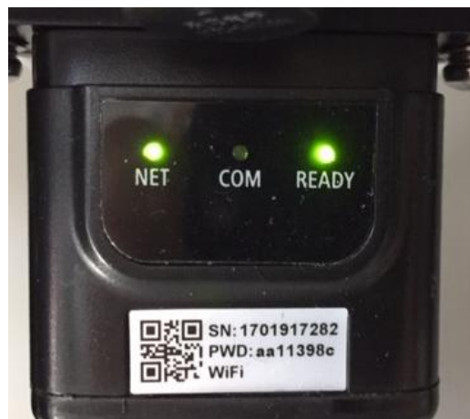
Figure 88 - Irregular communication status between the inverter and adapter
