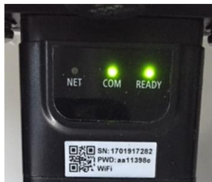
Figure 95 - Irregular communication status between the adapter and remote server
