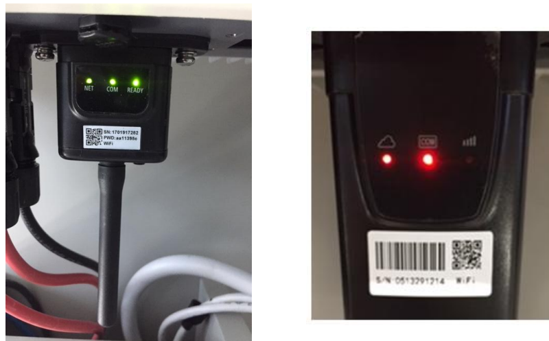
Figure 75 - Final status of LEDs
