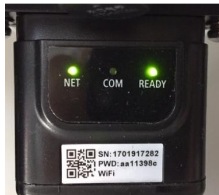
Figure 94 - Irregular communication status between inverter and adapter
