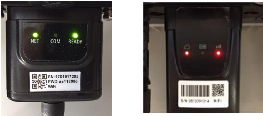
Figure 77 - Irregular communication status between inverter and Wi-Fi
