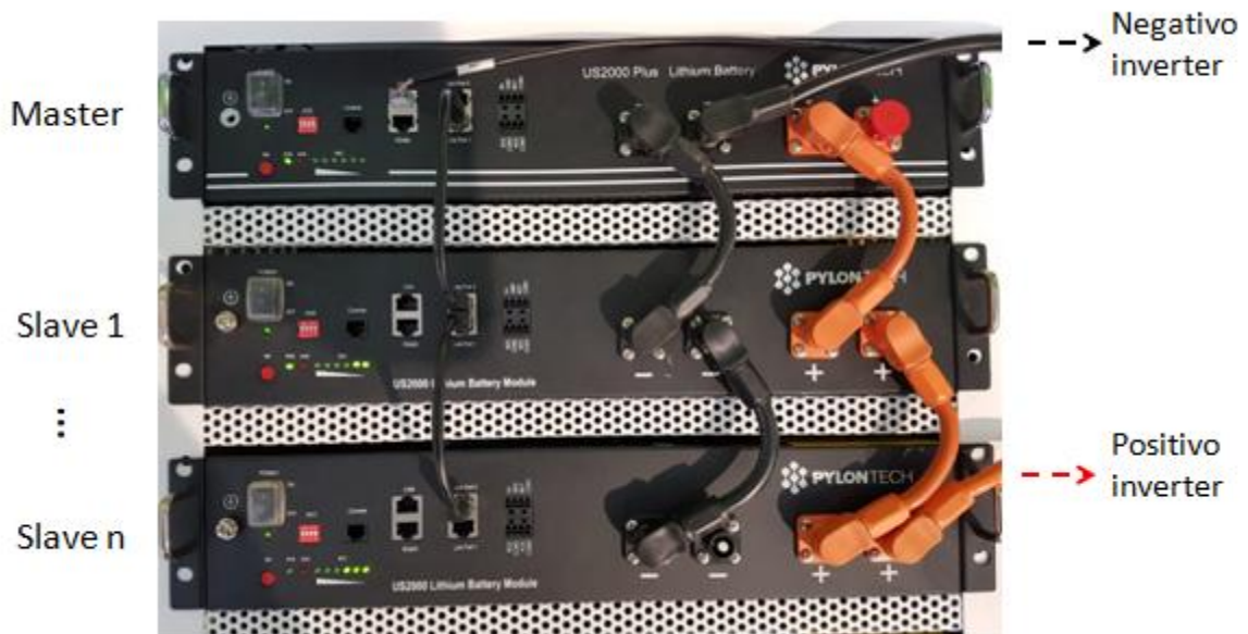
Figure 10 - Connecting three Pylontech batteries in parallel
