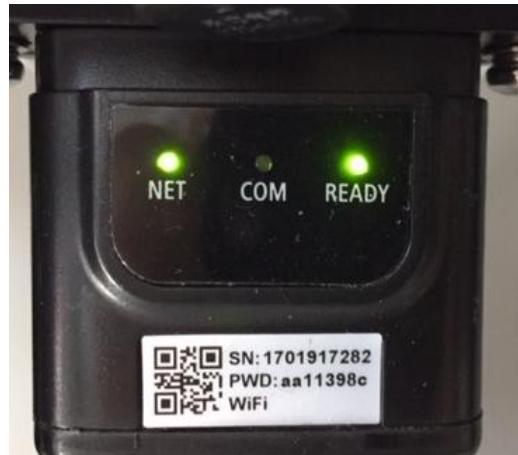
Figure 71 - Irregular communication status between the inverter and adapter
