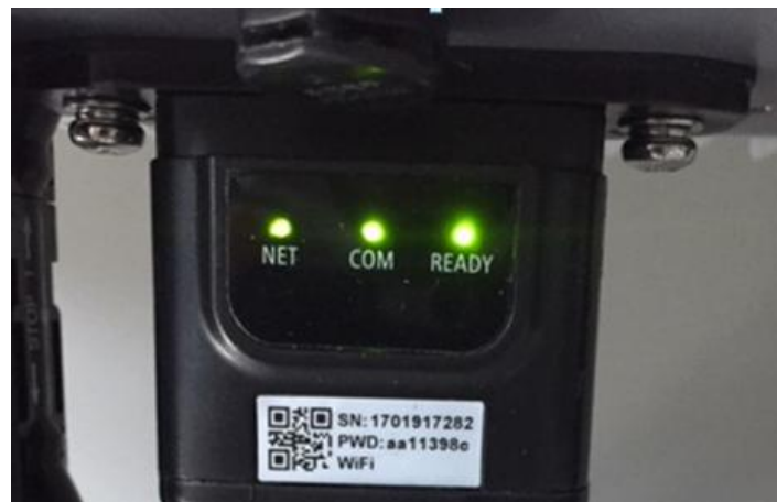
Figure 70 - Final status of LEDs
